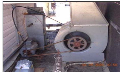
Two 5.5 kW heating, air circulation & moisture condensing system
